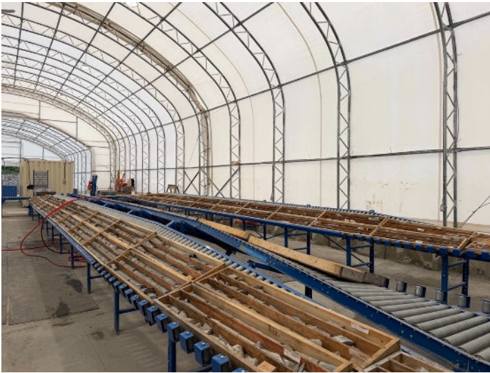
Exhibit 3 - Core Logging and Sampling Facility
